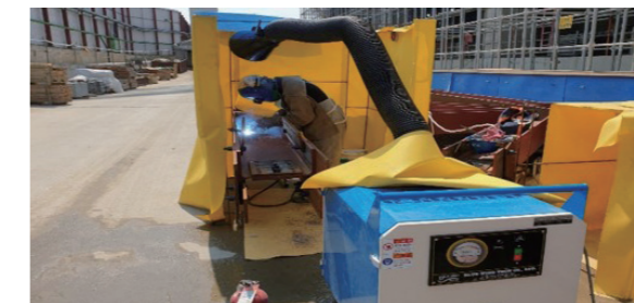
Installation of portable screen and dust collectors
